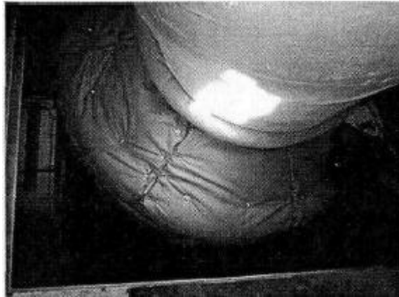
Insulation and protection of equipment
